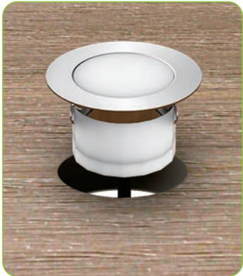
Step:2 Put the LED floor light into the hole
